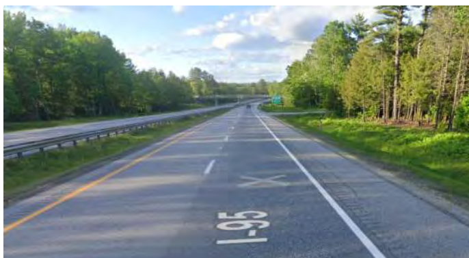
Photo 1: I-95 NB Near Poland Springs Bridge (2019)
