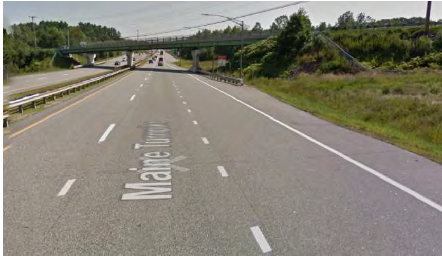
Photo 1: Just South of Exit 53 Southbound On Ramp
