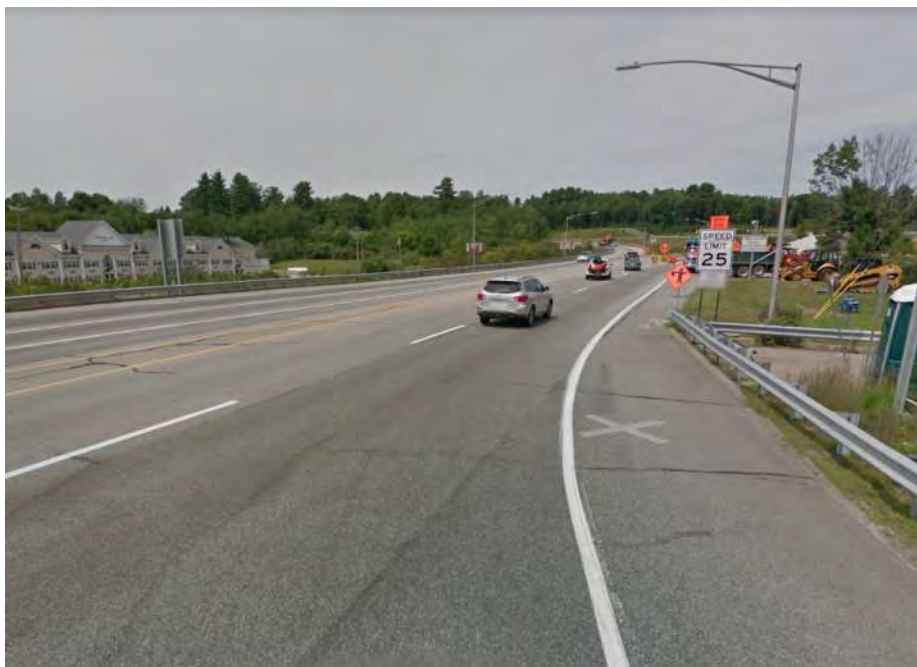
Photo 1: Exit 75 Ramps Weave (2018)
