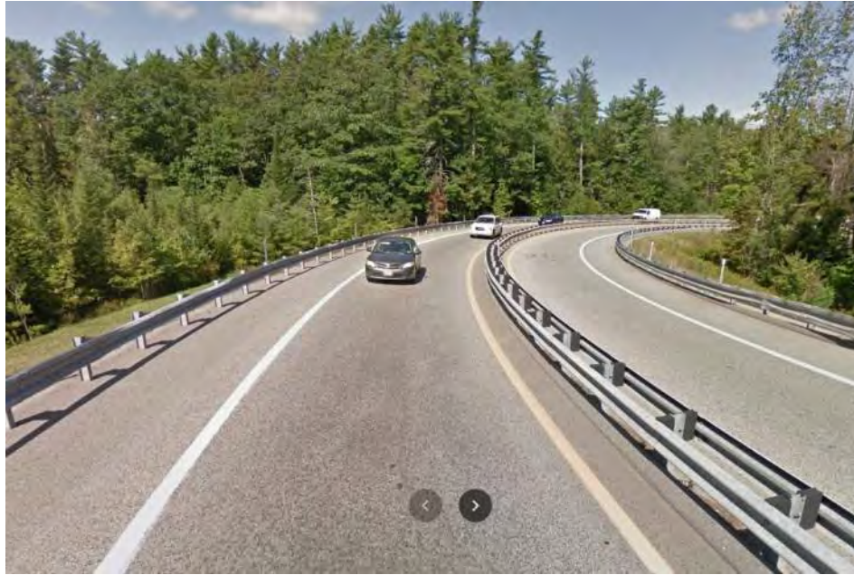
Photo 5: Exit 32 SB Off Ramp
