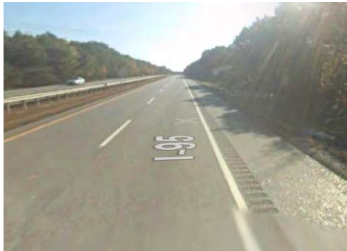
Photo 3: North of SB Toll Plaza (2008)
