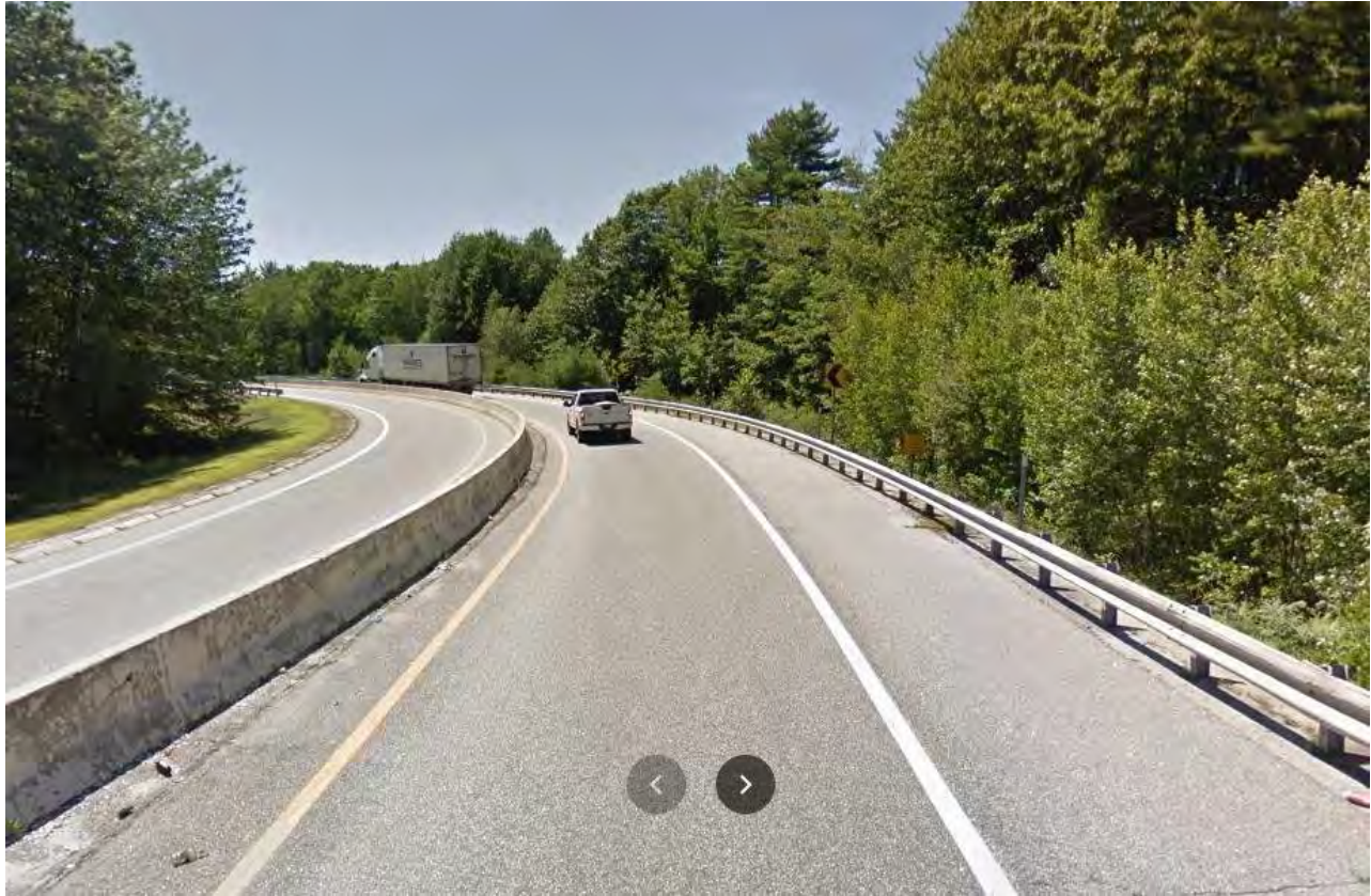
Photo 1: Exit 36 SB Off Ramp
