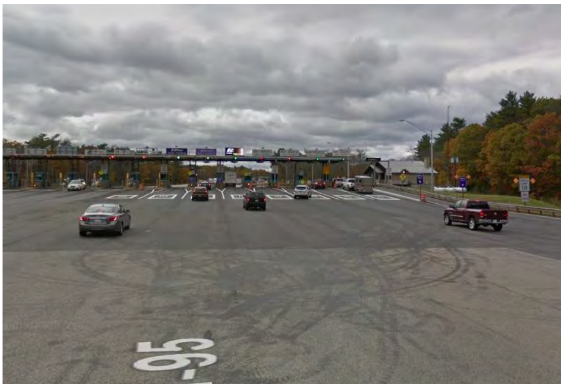
Photo 4: SB Toll Plaza (2018)
