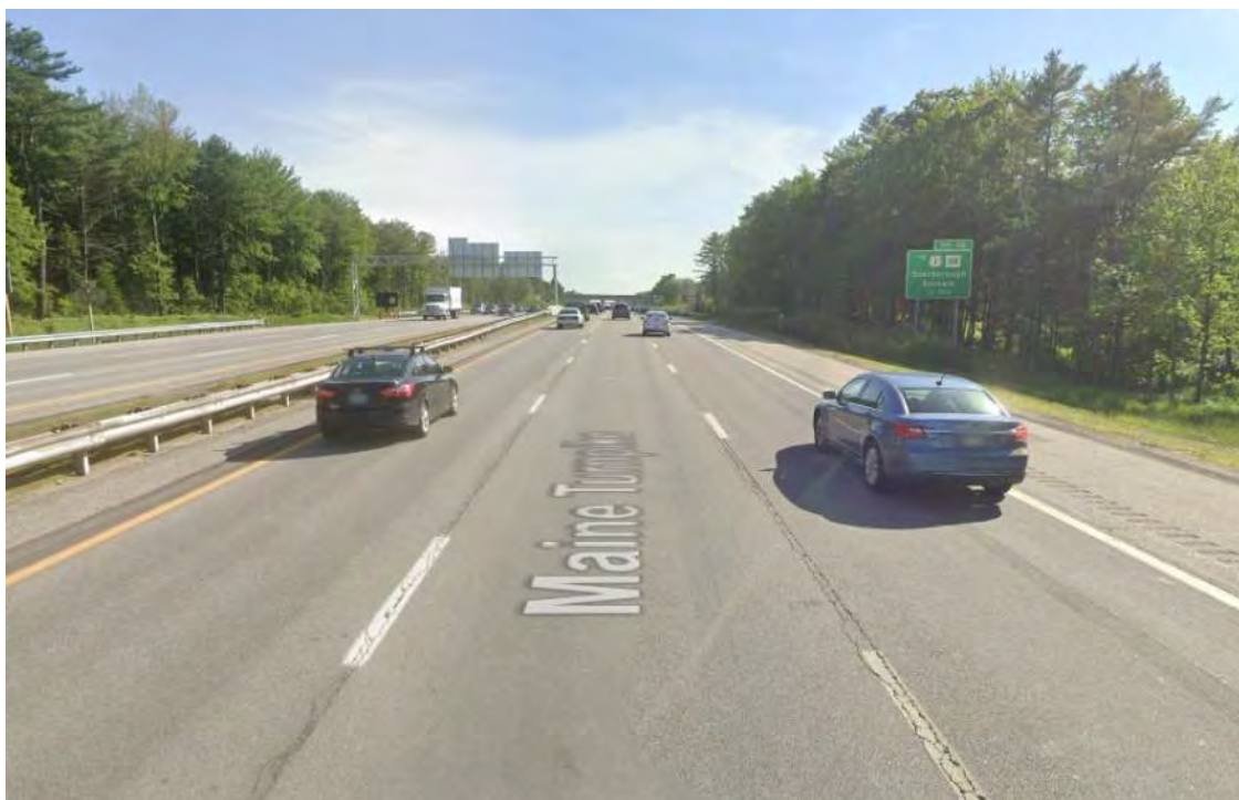
Photo 1: Exit 42 SB Off Ramp Approach
