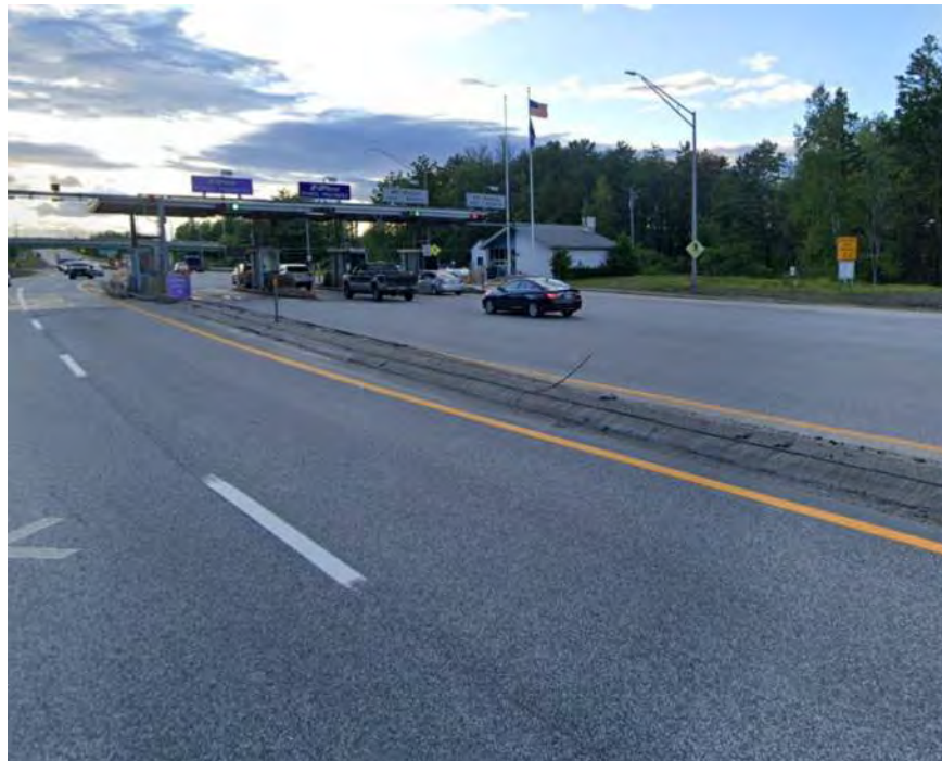
Photo 1: Exit 45 On Ramp Toll Plaza (2021)
