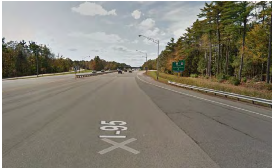
Photo 3: South of SB Toll Plaza (2011)
