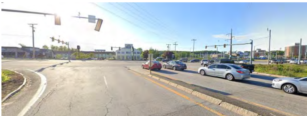
Photo 3: Exit 45 On Ramps Intersection (2019)
