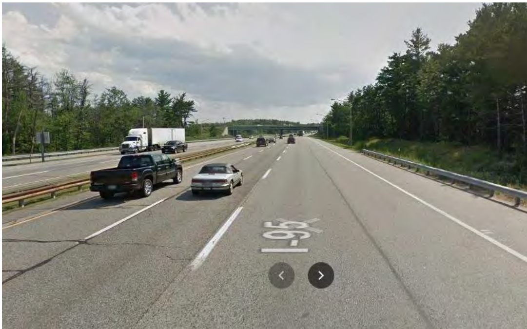
Photo 2: Segment after Exit 32 SB On Ramp (2011)
