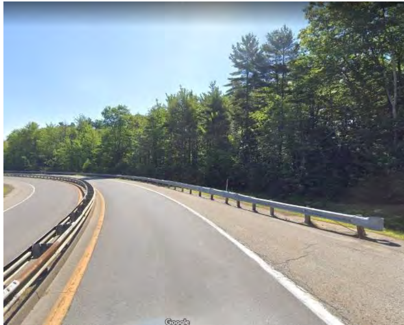
Photo 2: HCL 78 – Northbound On-Ramp
