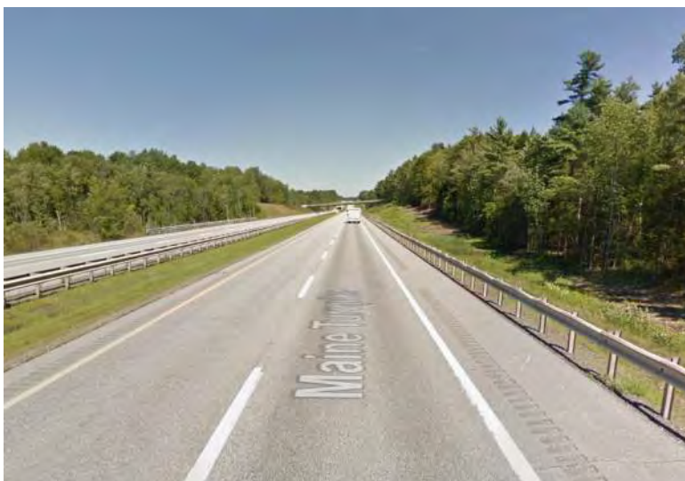
Photo 3: NB Segment Near Stevenstown Road
