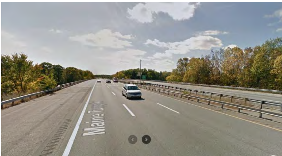
Photo 1: Mainline over Saco River
