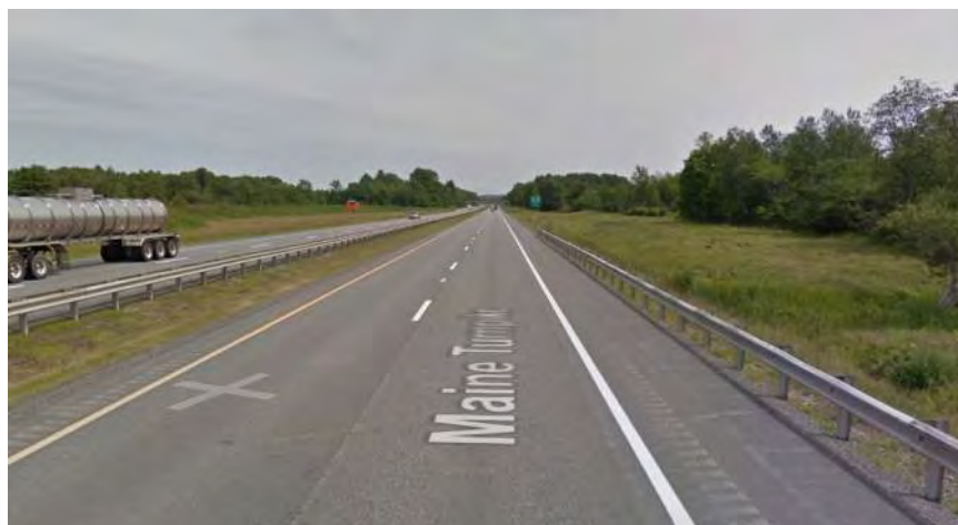
Photo 1: I-95 NB Near Grove Street (2018)
