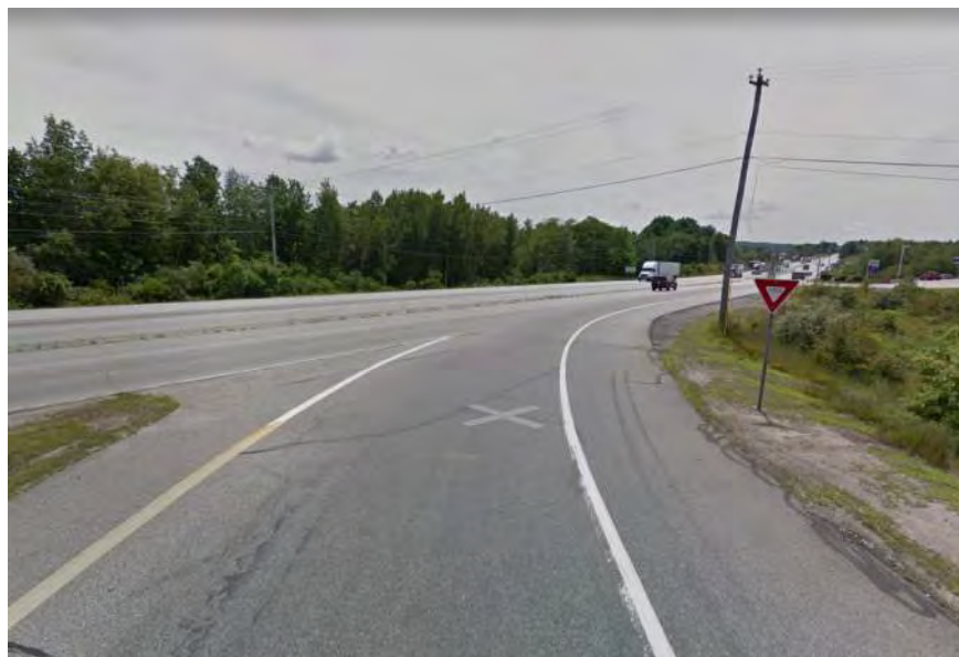
Photo 2: Exit 75 Off Ramps Slip Ramp Merge (2018)
