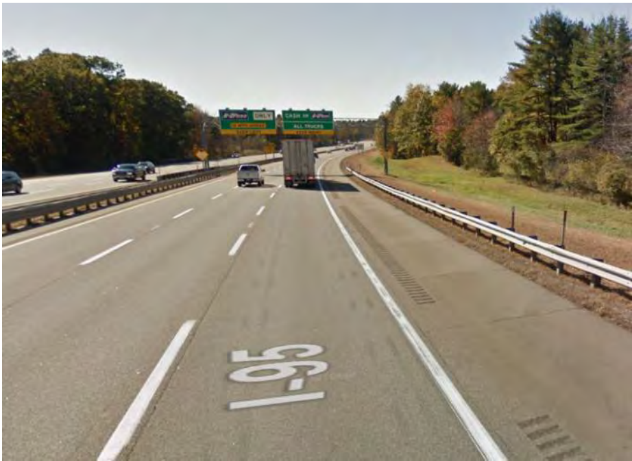
Photo 5: North of SB Toll Plaza
