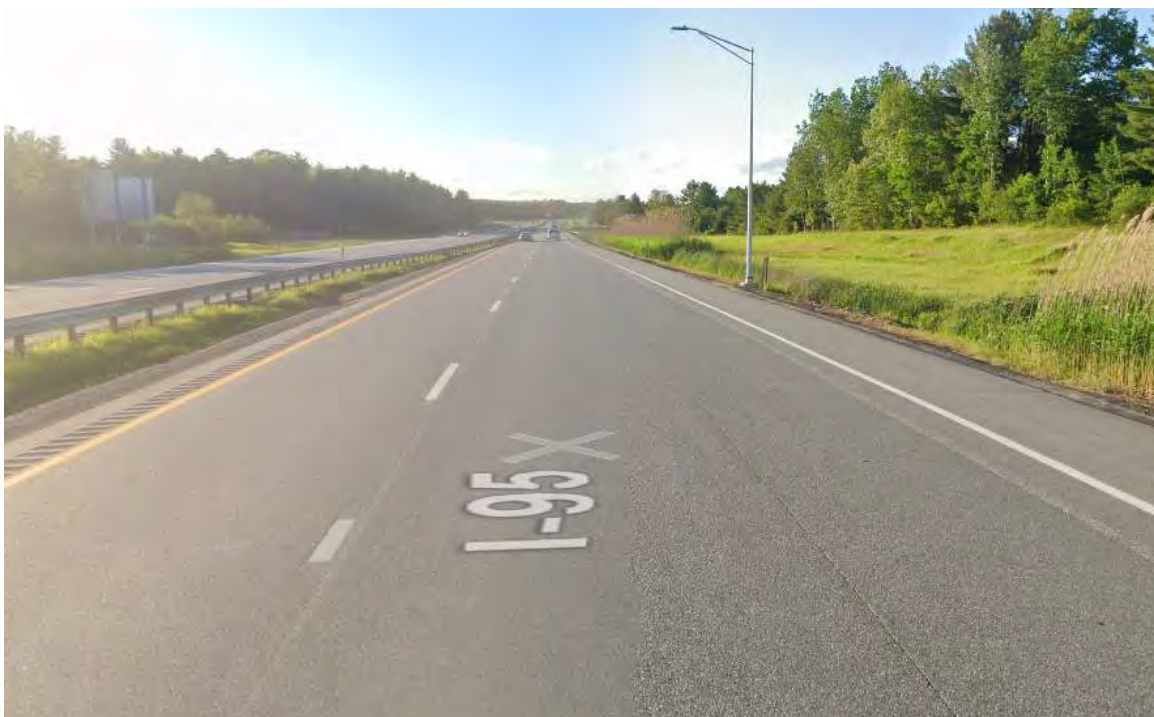
Photo 1: Just North of Exit 63 NB On Ramp (2019)
