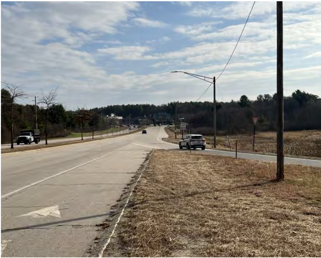
Photo 3: Slip Ramp Intersection from Spur Road (November 2022)
