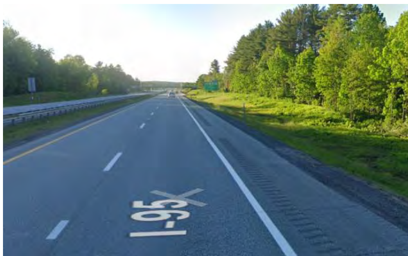
Photo 1: South of Exit 63 Off Ramp (2019)
