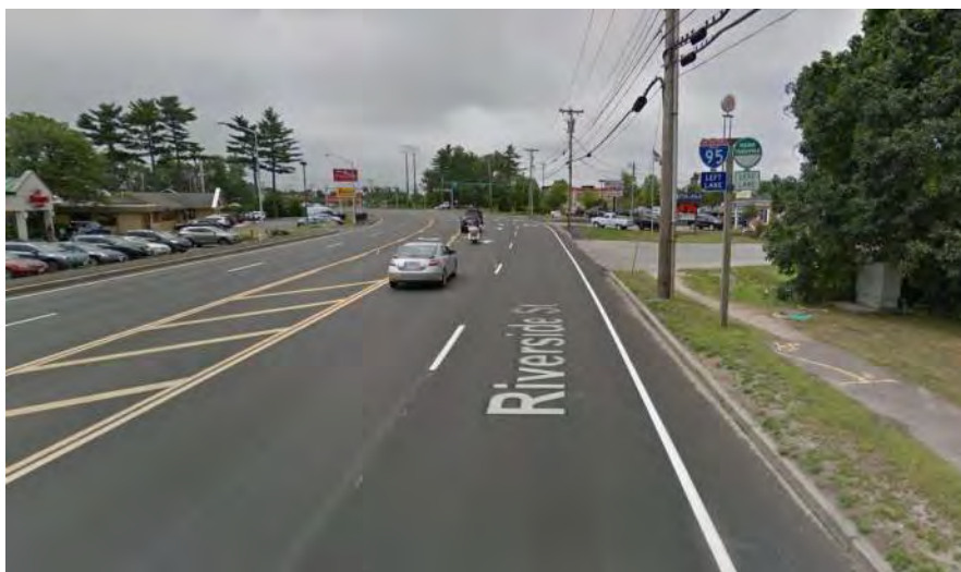
Photo 2: Riverside Street Southbound Approach (2018)
