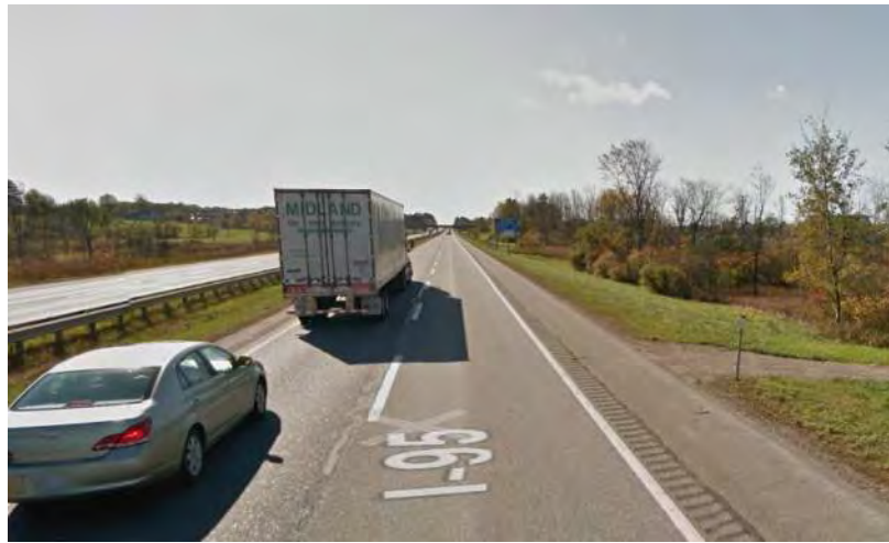
Photo 1: I-95 SB Just South of Exit 109 Interchange
