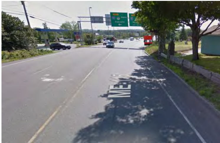
Photo 1: NB Ramps Intersection WB Approach (2018)
