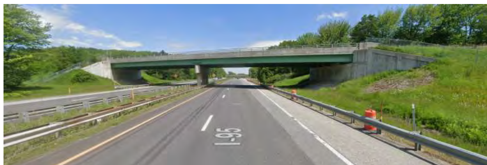
Photo 1: I-95 NB South of Exit 47 Off Ramp (2019)
