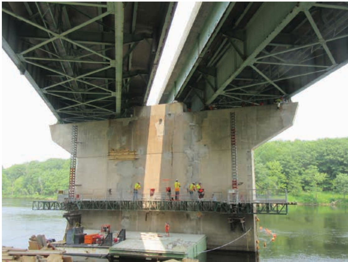
Androscoggin River Bridge Pier Rehabilitation, July 2019.
