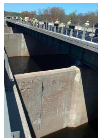
SACO RIVER OVERPASS DECK REPAIR AND RESURFACING
