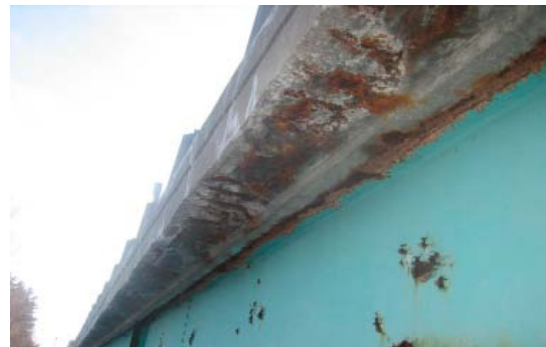
CENTRAL STREET BRIDGE OVERPASS
