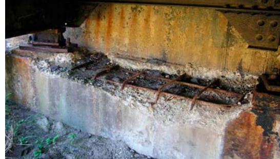
FURBUSH ROAD UNDERPASS
