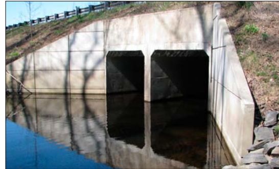
TWIN 8' x 8' CONCRETE BOX CULVERTS CARRY THACHER BROOK BENEATH THE MAINLINE IN KENNEBUNK
