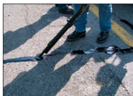
DISPENSED AT OVER 350 DEGREES THE RUBBERIZED ASPHALT SEALANT IS INJECTED DIRECTLY INTO THE PAVEMENT CRACKS
