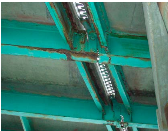
PIN-AND-HANGER ASSEMBLY AT THE YORK RIVER BRIDGE
