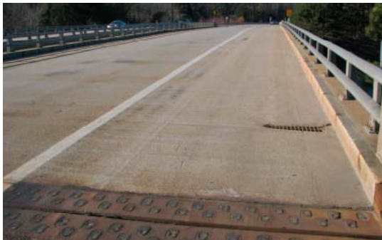
SACO INTERCHANGE BRIDGE
