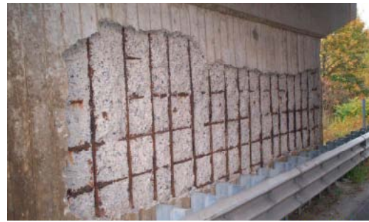
LEIGHTON ROAD UNDERPASS
