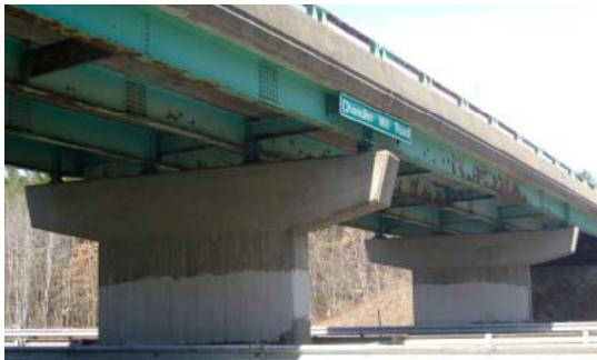
CHANDLER MILL ROAD UNDERPASS
