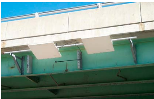
AUBURN INTERCHANGE OVERPASS
