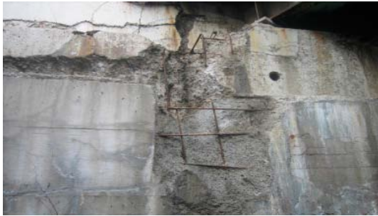
HUNTS HILL ROAD OVERPASS
