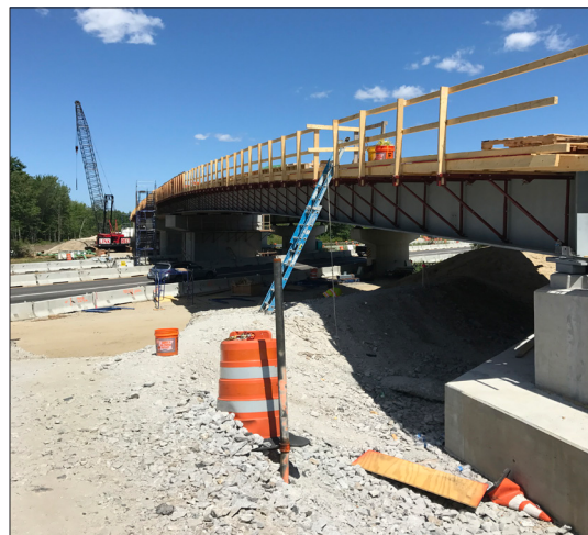
CUMMINGS ROAD UNDERPASS, MILE 44.6
