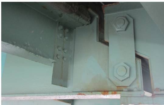
PIN-AND-LINK ASSEMBLY AT THE YORK RIVER BRIDGE
