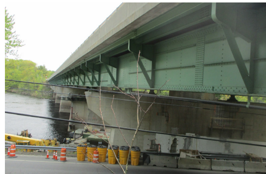
ANDROSCOGGIN RIVER BRIDGE
