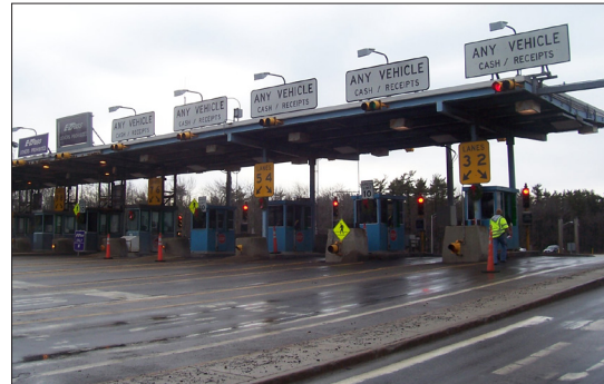
EXISTING YORK TOLL PLAZA - CONSTRUCTED IN 1969
