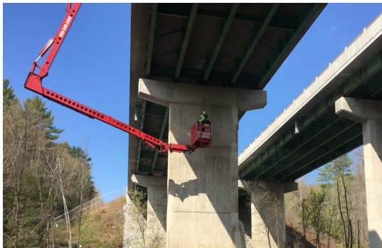
PRESUMPSCOT RIVER BRIDGE HANDS-ON INSPECTION
