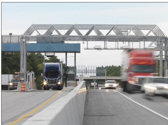
NEW GLOUCESTER TOLL PLAZA
