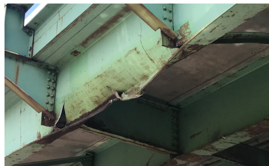
SOUTH PORTLAND INTERCHANGE UNDERPASS, MILE 44.9
