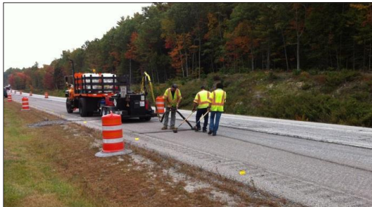
DISPENSED AT OVER 350 DEGREES THE RUBBERIZED ASPHALT SEALANT IS INJECTED DIRECTLY INTO THE PAVEMENT CRACKS
