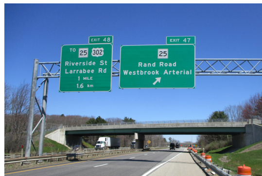
OVERHEAD SIGN BRIDGE MAINLINE NB, MILE 47.0
