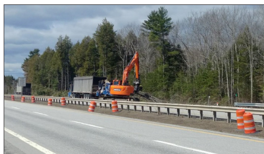
SIDE SLOPE CLEARING
