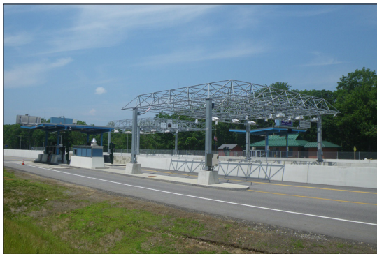
FALMOUTH SPUR TOLL PLAZA
