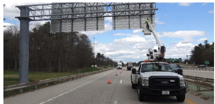
OVERHEAD SIGN STRUCTURE INSPECTION
