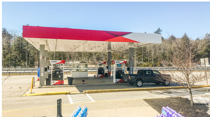
KENNEBUNK SERVICE PLAZA FUEL SYSTEM
