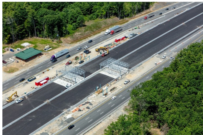
REPLACEMENT YORK TOLL PLAZA
