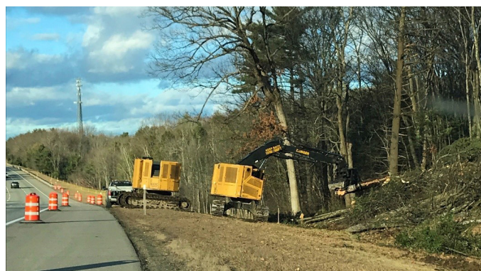
SIDE SLOPE CLEARING
