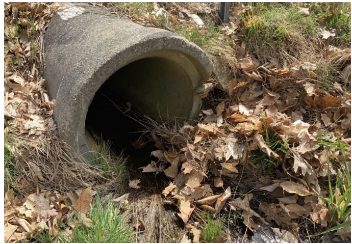
ROADWAY DRAINAGE CULVERT
