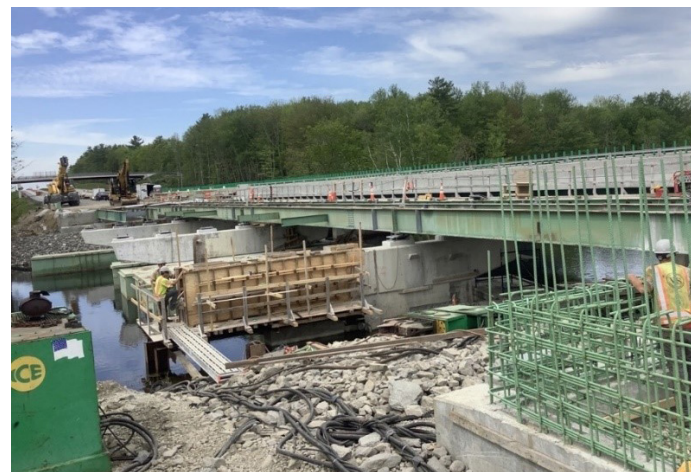
COBBOSSEECONTEE STREAM OVERPASS (NB) MILE 99.2
