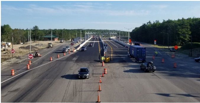
WEST GARDINER I-295 TOLL PLAZA REPLACEMENT
