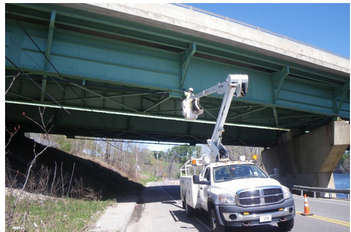
HANDS-ON INSPECTION OF THE ANDROSCOGGIN RIVER BRIDGE
