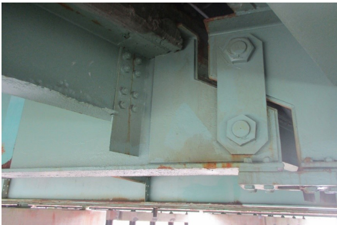
PIN-AND-LINK ASSEMBLY AT THE YORK RIVER BRIDGE
